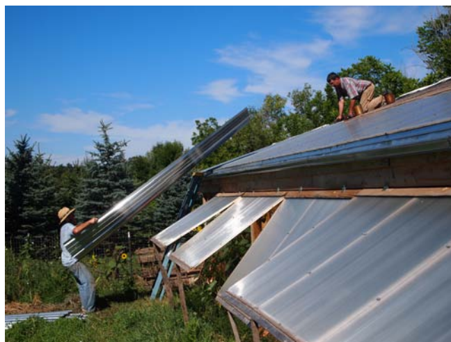
removing the roof, 96 degrees
